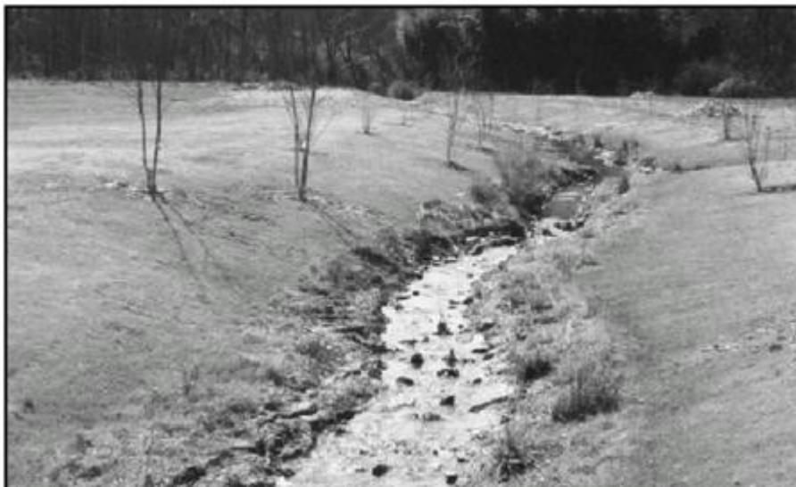
One year after restoration, the stream has taken to its new channel-reshaped channel in the foreground, daylighted channel in the background (picture courtesy of DeKalb Parks Department).
